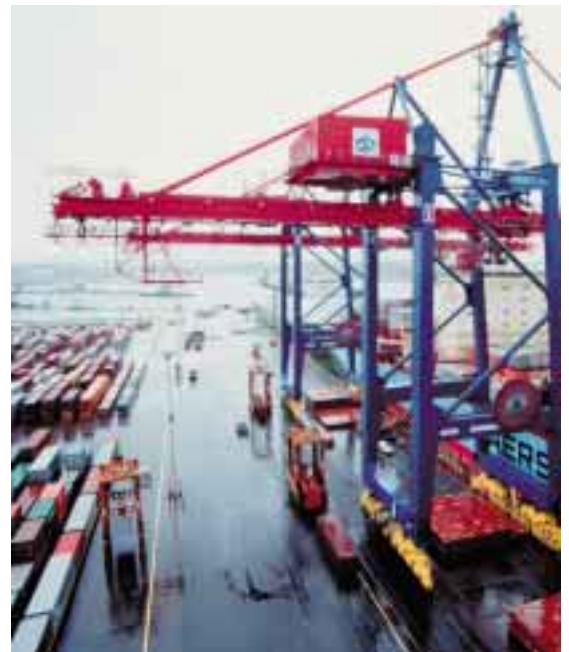
With the advent of containerisation, transshipment of goods between the modes has become a faster and more cost efficient operation. Today, the container crane driver can move more than 700 tonnes of goods ship to shore in an hour.
