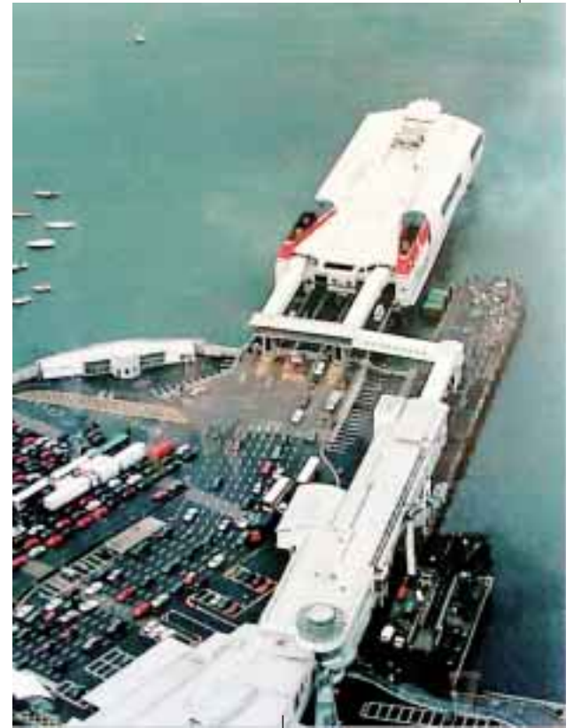
T he Stena Line terminal in Dun Laoghaire represents a specialised and very efficient HSC facility.
