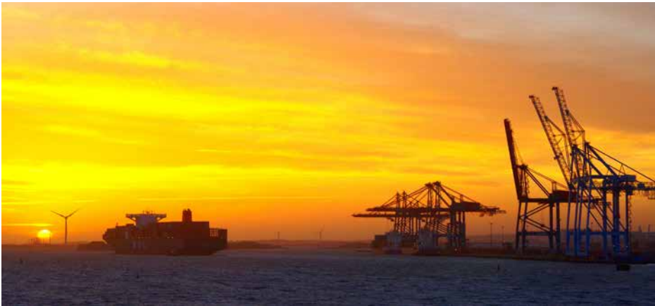
The demanding 24-hour operation of vessels. Photo courtesy of Lars Markström.
